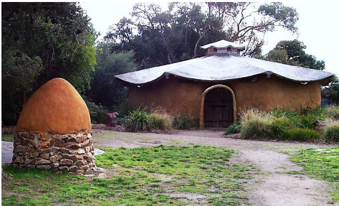
Figure 1. The hut and pizza oven built by HOL teams at Frankston High School.
